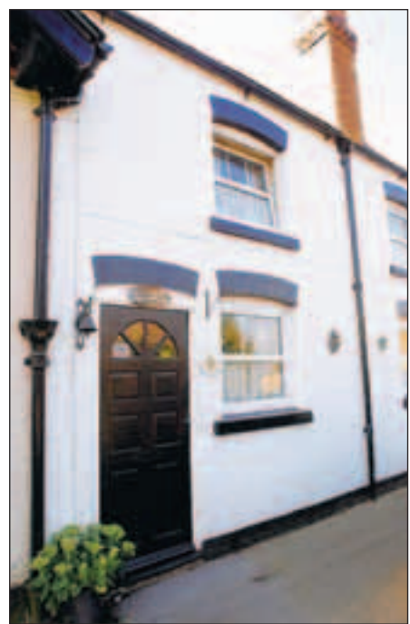
The fairly ordinary exterior of the Day's property hides a 1940s interior
