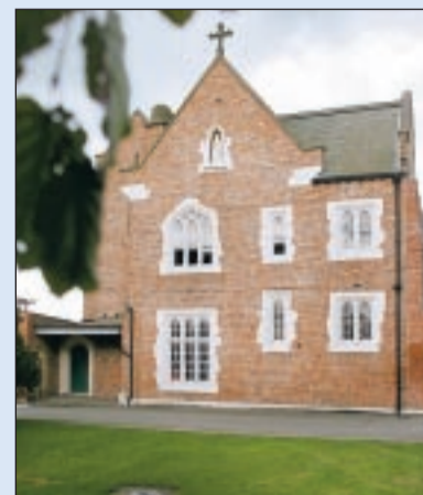
PURPOSE-BUILT: Gratia Care
