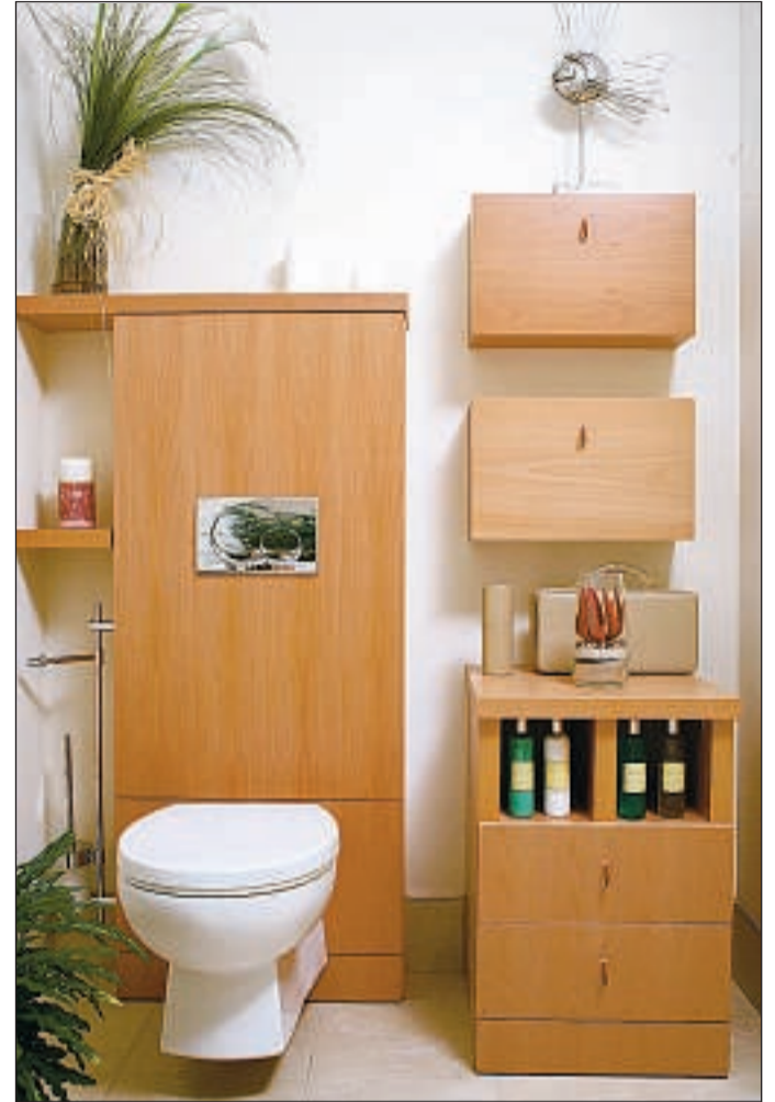
PIPE-FREE ZONE: Michelle and Graham's stunning bathroom has been designed to hide away unsightly plumbing
