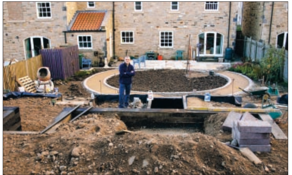
ADDING STRUCTURE: Ian Lamming surveys the ongoing works
