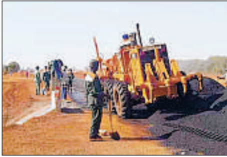
Road construction can lead to problems
