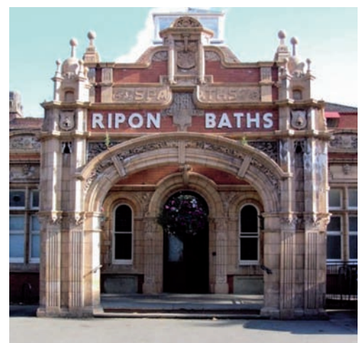
Ripon Baths, where the row over the historic building goes on
